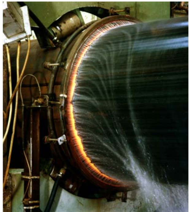
Figure 2: Detailed view on induction coil and heated zone during bending
